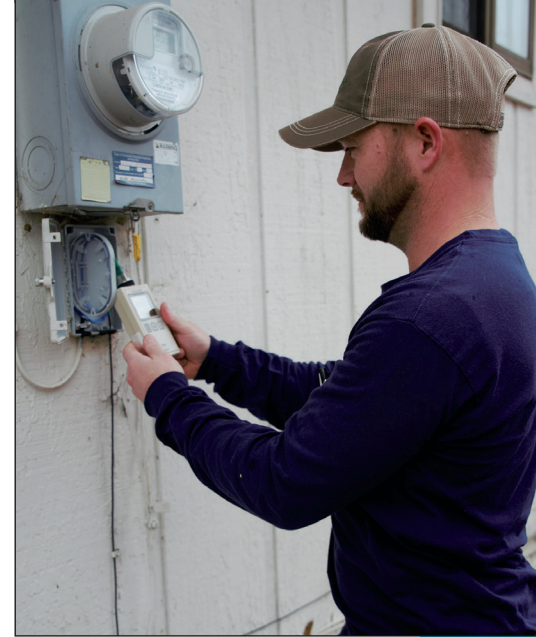
Gibson Connect Installation/Repair Tech 1 Zach Elliott tests the light level before starting an installation.
